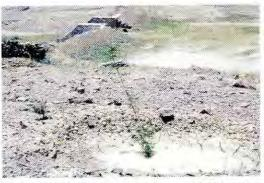
More than 1200 eyebrow pits were excavated along the contours in staggered fashion to harvest the runoff water and to detain the silt load which accompany the runoff. Similarly, 40 trenches having the size  $10 \times 4 \times 2.5$  ft were excavated along the contours on the upslope steep hilly area of the catchment in an alternate manner to arrest the sediment and gravels coming with runoff.
